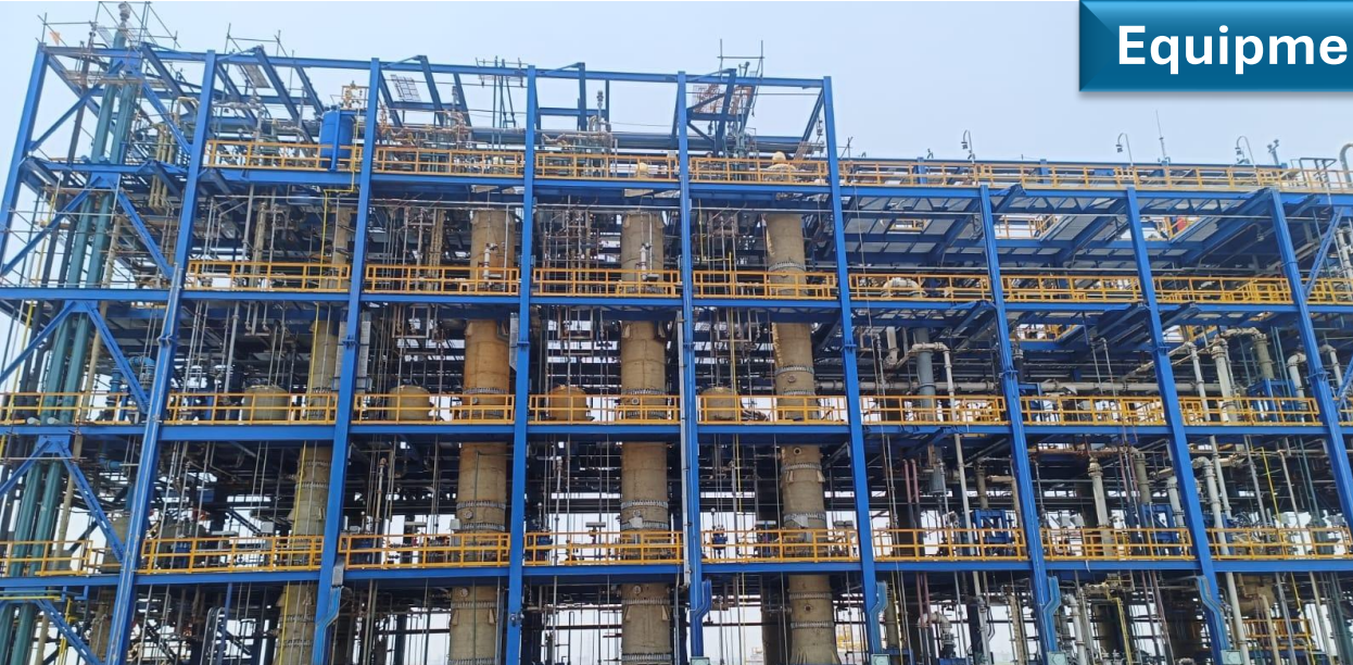
Column erection with inside silicon packing at GACL, Dahej
