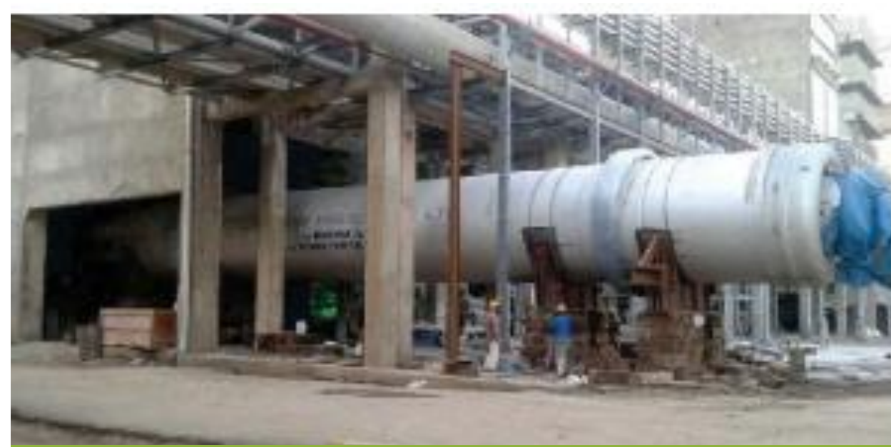
Horizontal Calciner erection at Nirma, Bhavnagar
