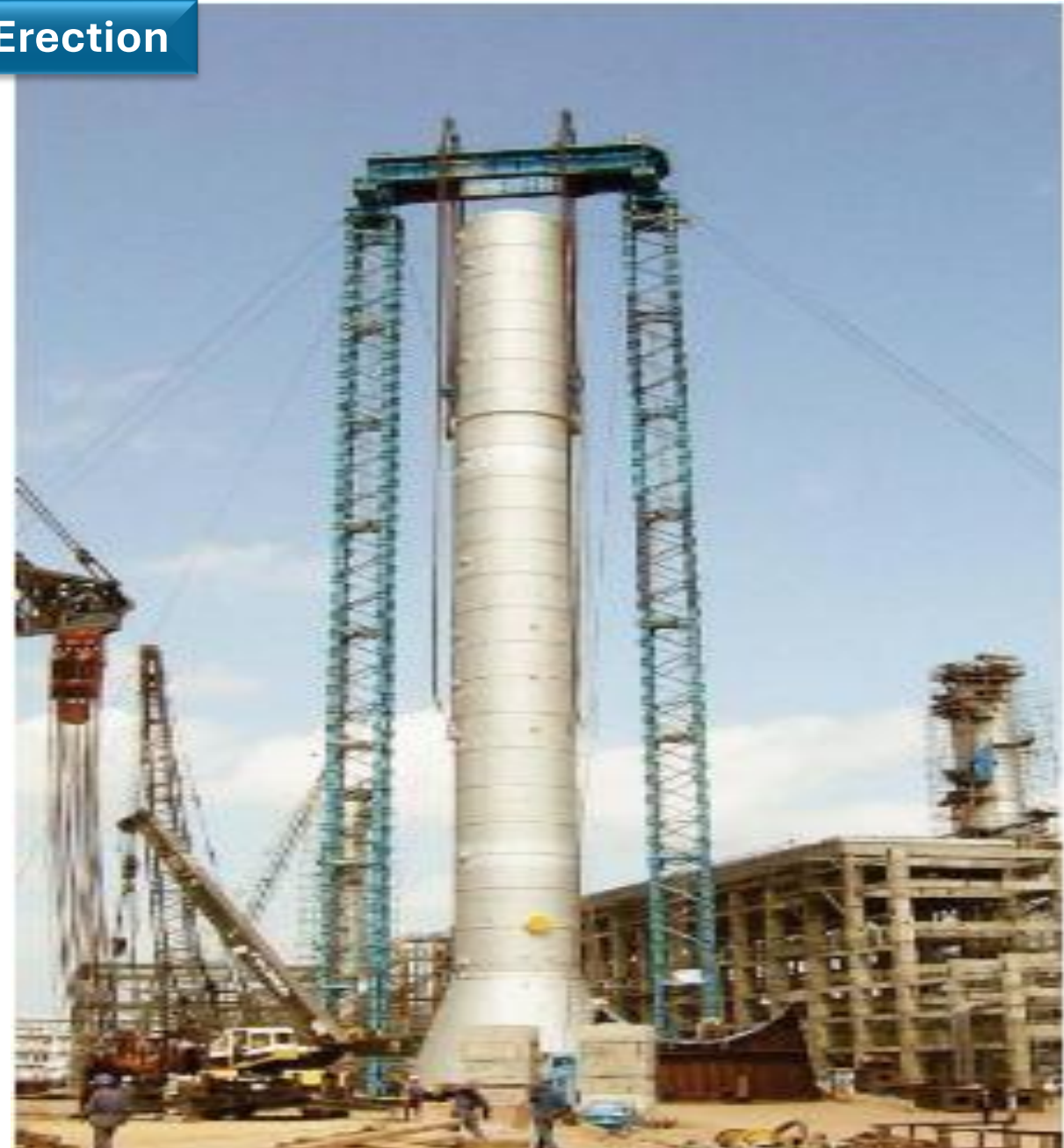
Fractional Distillation Column Single Piece Erection – Reliance, Jamanagar
