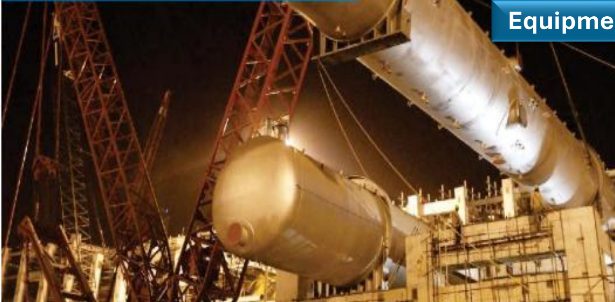
Column erection at Reliance, Jamnagar, GJ
