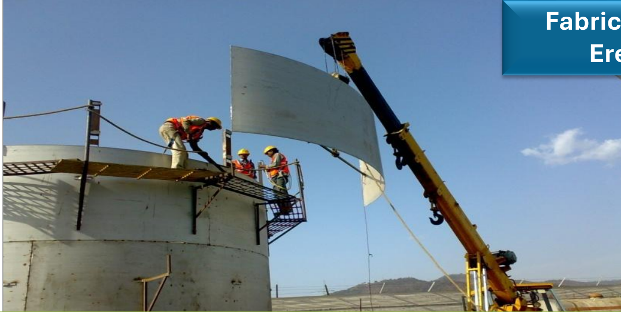
SS Tank fabrication at P&G, Mandideep, MP
