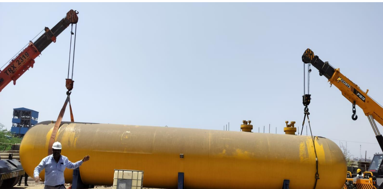
Nitrogen Bullet erection at GACL, Dahej
