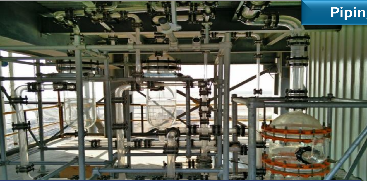
Glass Piping at Bromine Plant at Nirma Bhavnagar
